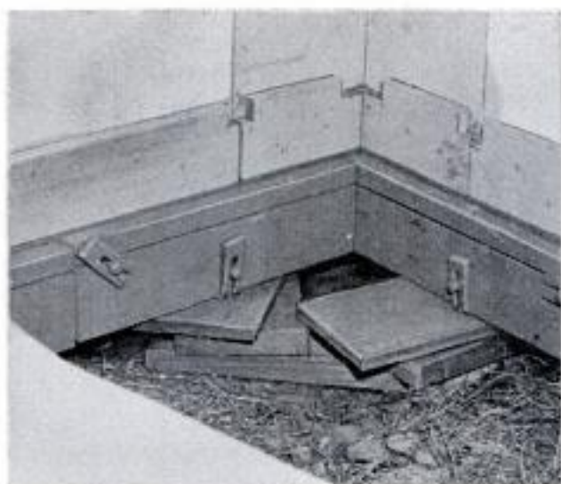
Bolts slip through predrilled holes and are held firmly with locking pins. Flooring is of plywood
